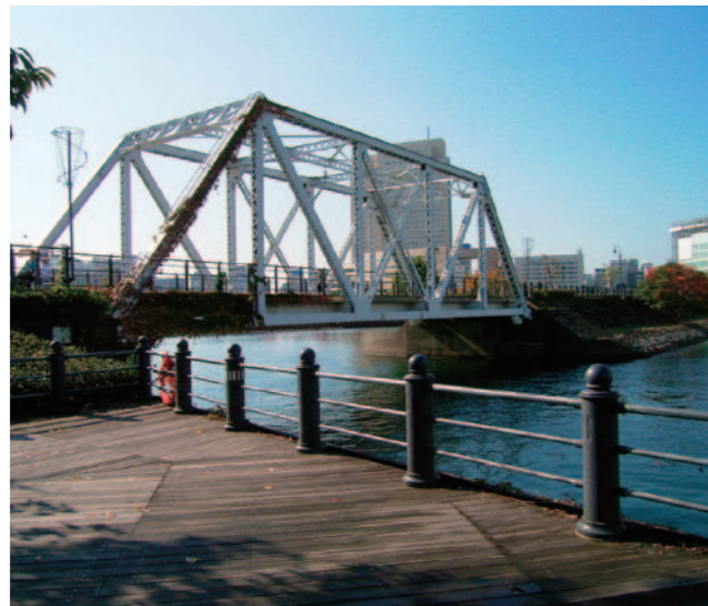
"Kisha-Michi" Promenade where three bridges and an embankment remain
